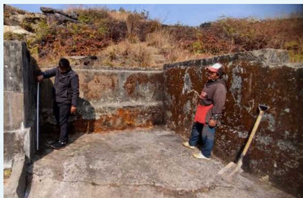
Site instruction for operation of open limestone channel (OLC) at Laitryngew, Shella block under MLAMP.
