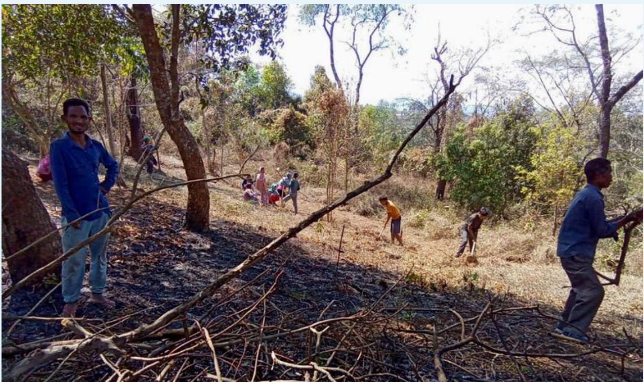
Preparation of land for construction of Community Hall at Chandigre under Rongram land
