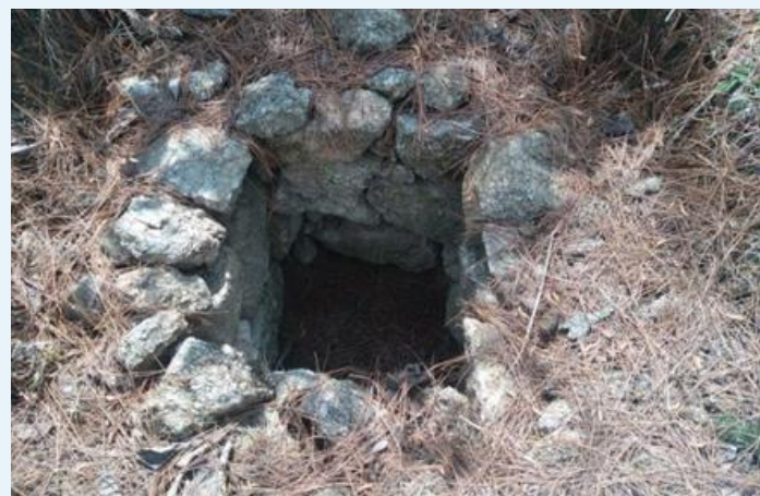
Inspection of recharge pit at Lai Kyntoit under Myllichem Block
